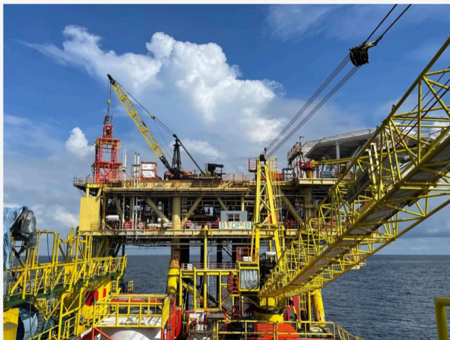
Offshore CTU Well Intervention Project Supported by Thunder Cranes
